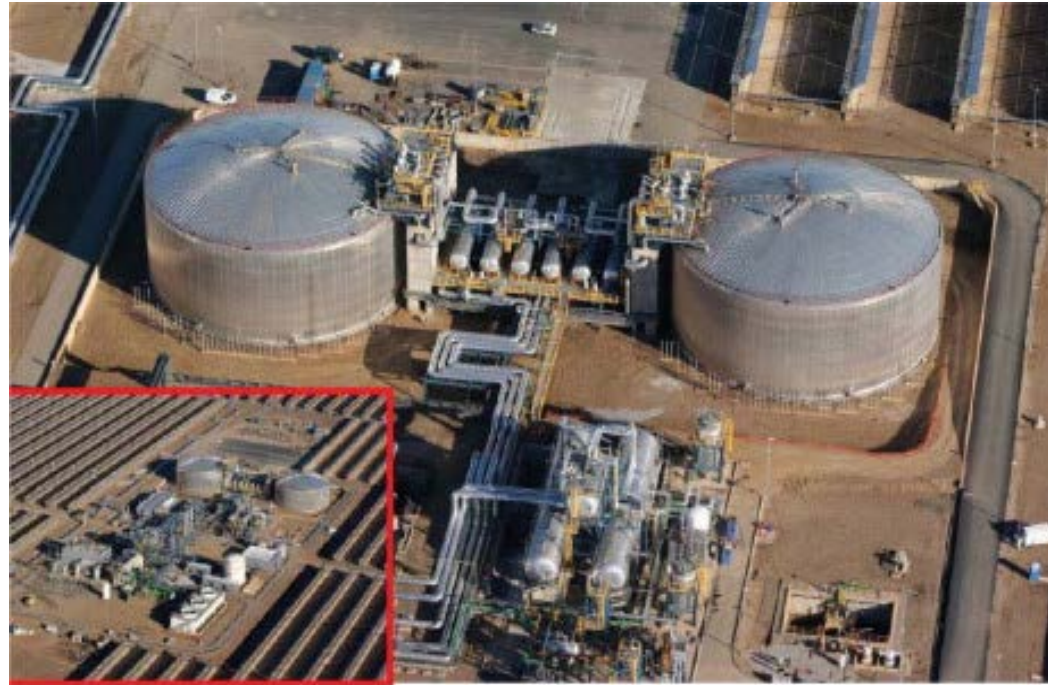
View of a 2-tank molten salt heat storage system
