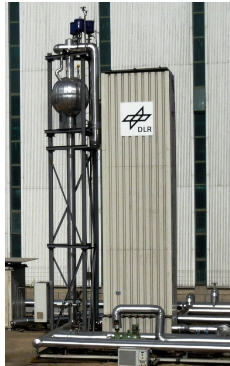
700 kWh PCM prototype (Project REALDISS)
