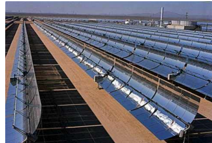
View of a typical solar field
