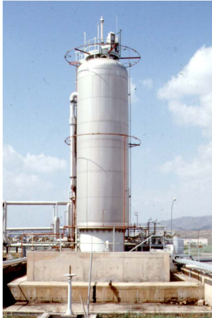
Thermocline storage tank at PSA
