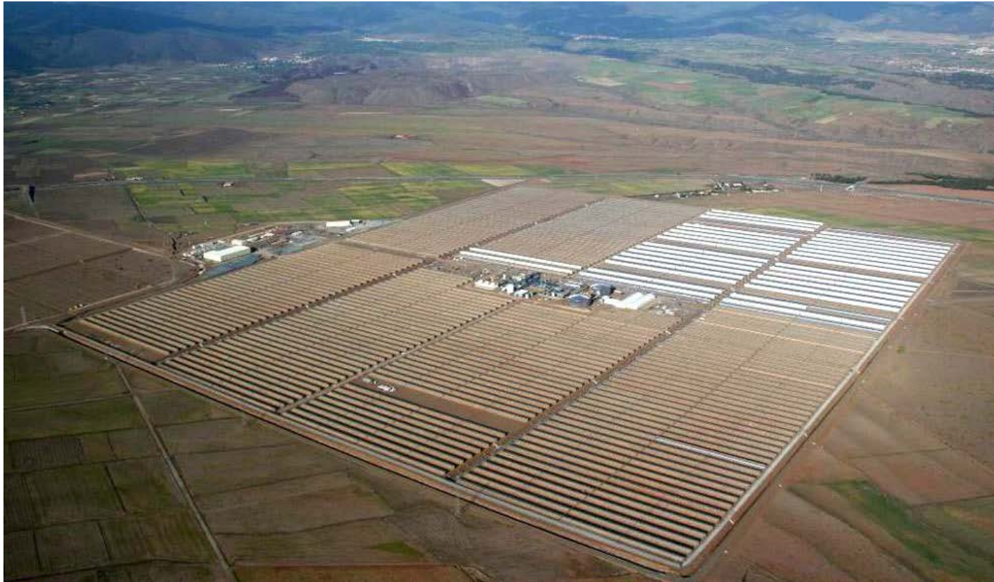
Aerial view of the 50 MWe ANDASOL-I plant
